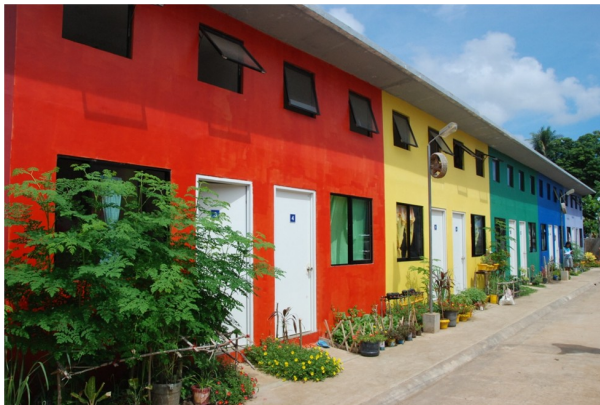
Housing units at SM Cares Village Bogo Cebu
